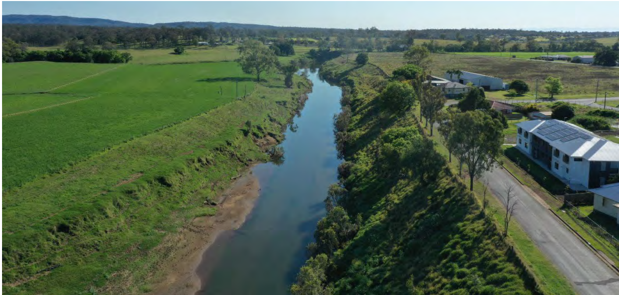
Figure 8. A contraction reach of Lockyer Creek near Gatton. The floodplains are rarely inundated, and flows are largely contained within the channel leading to high rates of channel erosion and limited floodplain deposition
